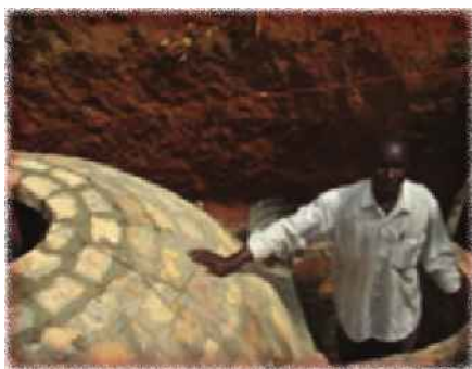
Biogas unit under construction in Kakindu Subcounty
